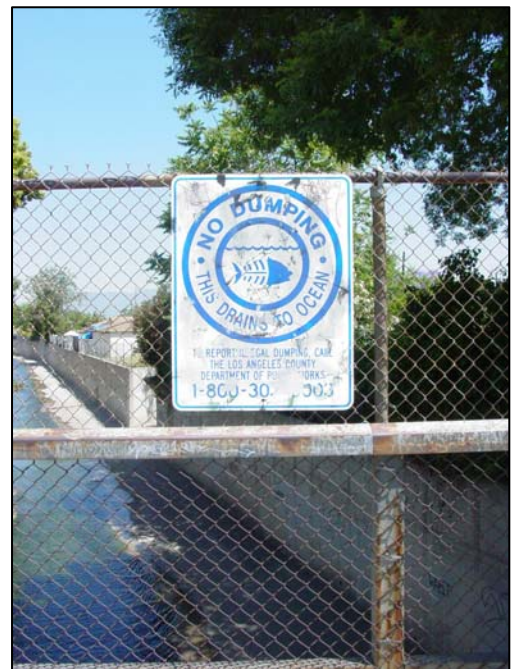
No Dumping Sign along the Rio Hondo Flood Control Channel
