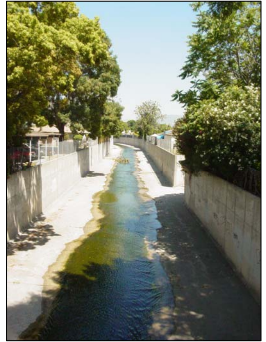
Cemented Rio Hondo flood control channel
